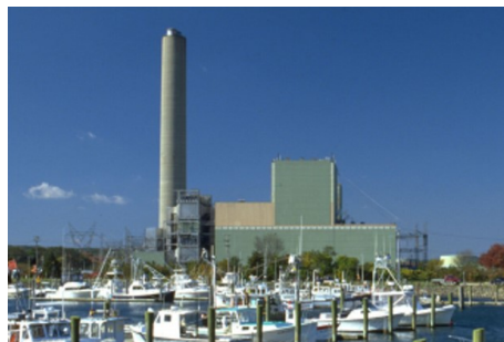
Canal 2 plant (Source: NRG Energy)
